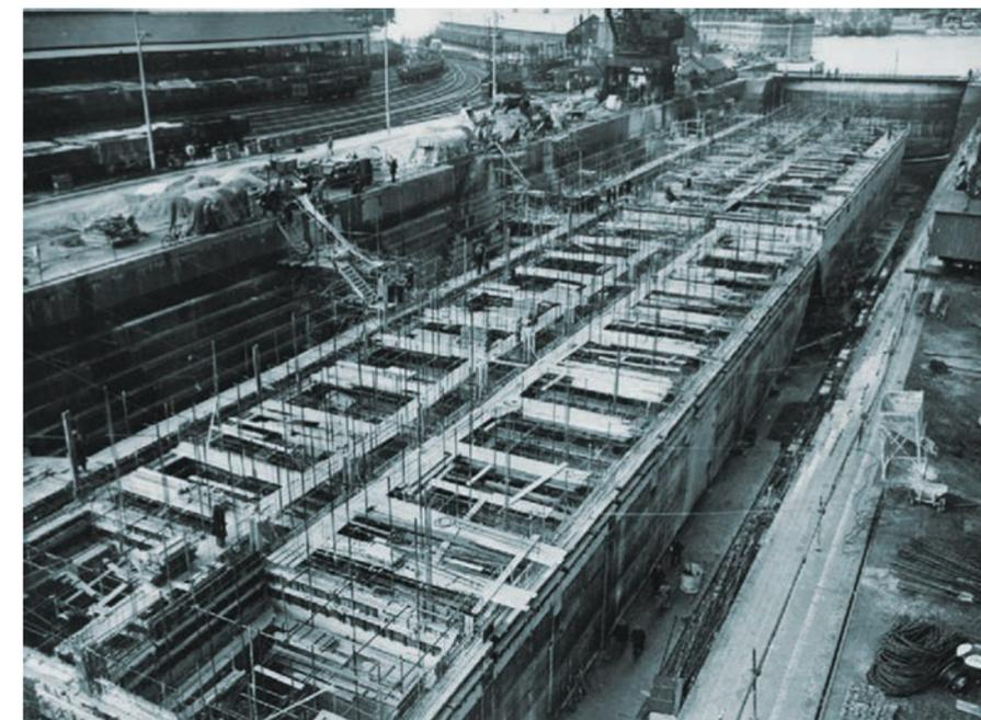
**Concrete caissons for the main breakwaters were typically constructed in two stages. Workers would first build the lower part in a dry dock, above, then launch it and erect the remainder of the structure from inside the caisson itself. Some of the floating bridge spans, below, could be lengthened or shortened to accommodate the tides.**
