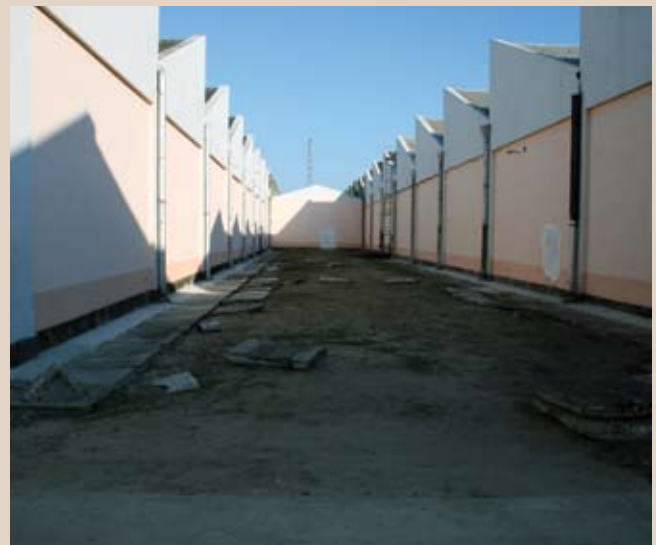
Previously a textile factory, Transcom Sharaf's warehouse is now fully tobacco compliant.
