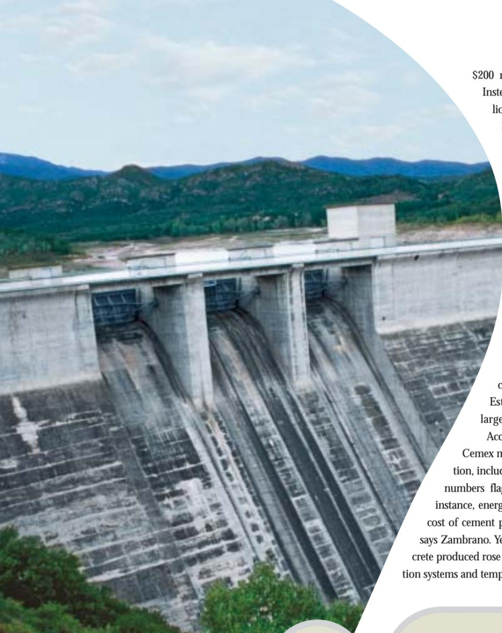
WHEN COMPLETED, THE EL CAJON DAM WILL CONTAIN MORE THAN 21 MILLION CUBIC FEET OF CONCRETE.
